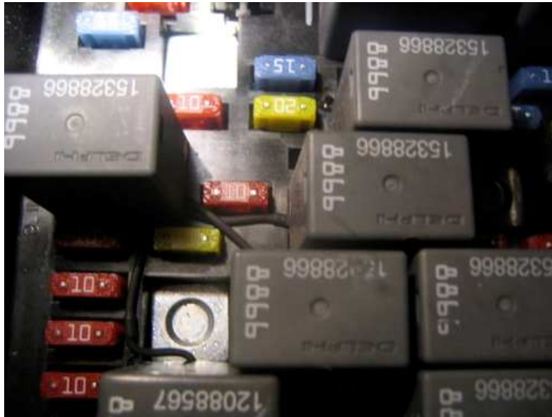
Pic 11 – All diodes run and relays installed
