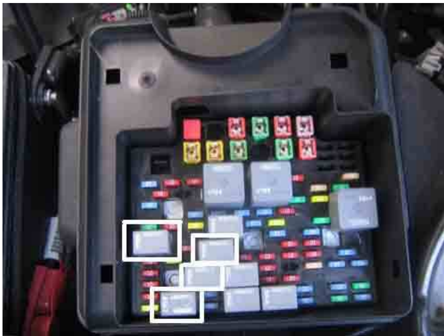
Pic 6 – Relays highlighted with white box
