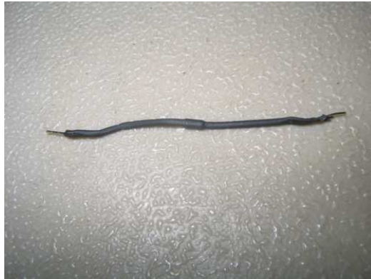
Pic 3 – Heat Shrink applied
